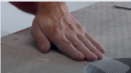
1 Place Skamol Joint Tape.
