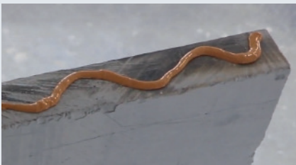
1 Reinforce SkamoEnclosure Board joints, using Skamol Glue.
