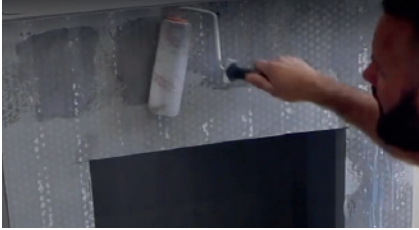
1 Forbered SkamoEnclosure Boards.
